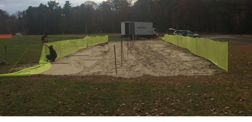
Typically 6-8 inches should be driven in and 1-3 inches of post should extend beyond the top of the fence. Enough post should be exposed so the fence can be hung at full height, but avoid leaving excessive height above the fence. In some situations a row of course tape can be strung parallel to the fence using the tops of each stake to increase branding opportunities and clean up extra post space.
